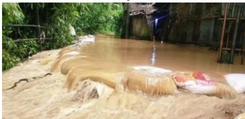
Figure 8: A breach in the Kushiara River embankment in Zakiganj, Sylhet, caused by heavy rainfall and upstream flows. (Source: Dhaka Tribune , June 2, 2025).
