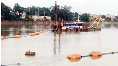
Figure 9: A dredging project on the Surma-Kushiyara river system designed to reduce siltation and mitigate flooding. (Source: Voice7 News, August 6, 2025).
